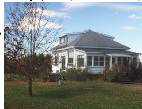
The fourth (or new) Marlinton school located between chemins Lamarche and Davis. It is now a private residence.
