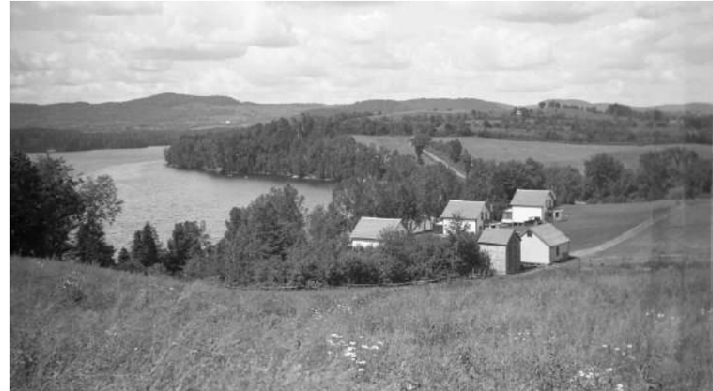
Three of an eventual six rental cabins built for Armand Houle at Harvey Bay, as seen in the late 1930s. Purpose built rentals faded by the 1960s. Image courtesy of Gilbert Elliott.
